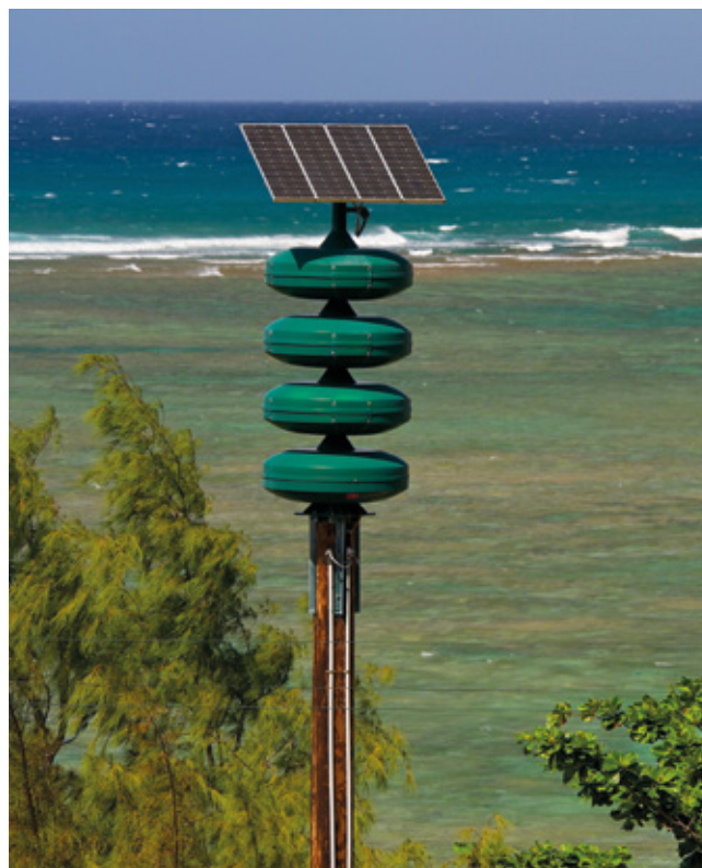
Tsunami Warning Tower, Pacific Islands
