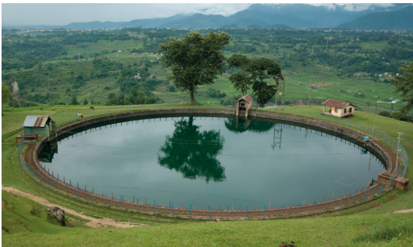
Small water reservoir for Hydroelectric Power, Nepal
